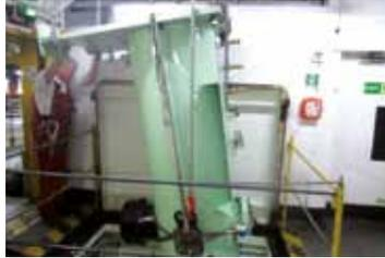
Condenser rigging through access hatch.
