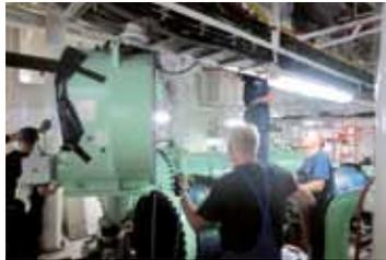
Condenser fitting through watertight door. Chiller being reassembled in machinery space.
